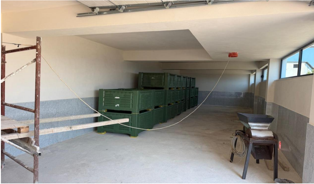
Figure C-3. Existing premises – representative internal view. Source: Berat Feasibility Study. Indicative – not for construction.
