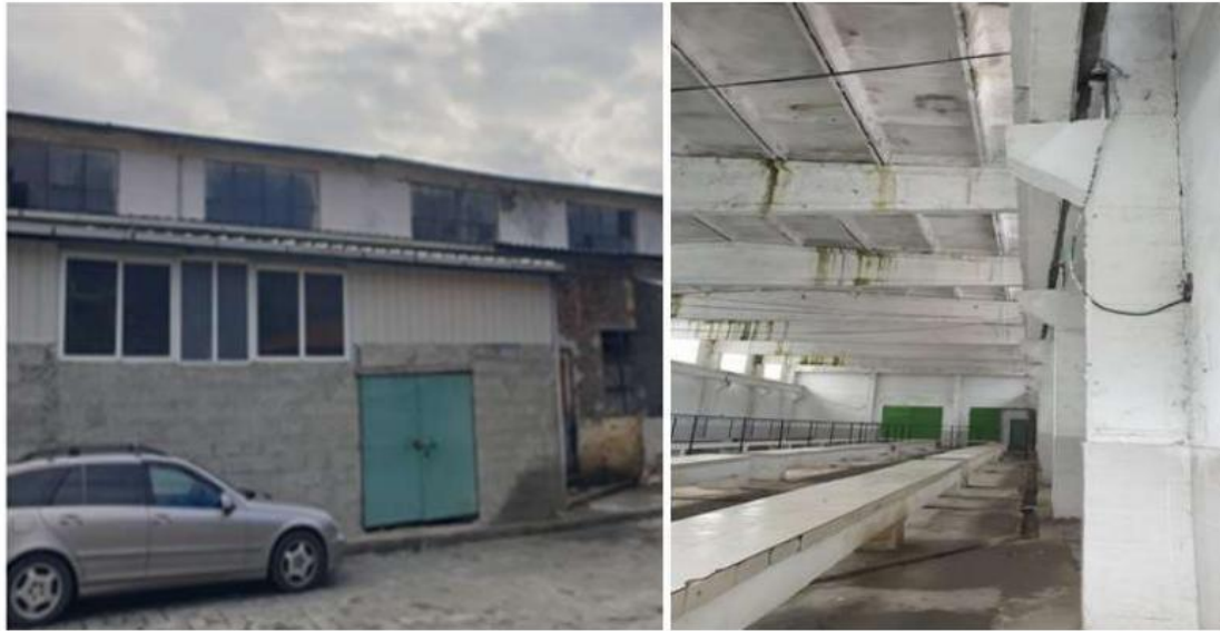
Figure 2.1 Existing Building – General View
